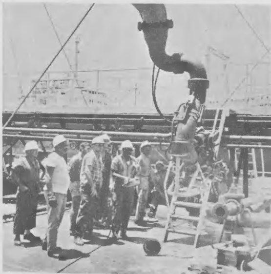
Oil Movts. Shift Foreman Julian Daniel (Picture left & right) shows how to operate control box to hook up metal loading arms. In center is a hydraulic coupling device to connect on tanker flange.
